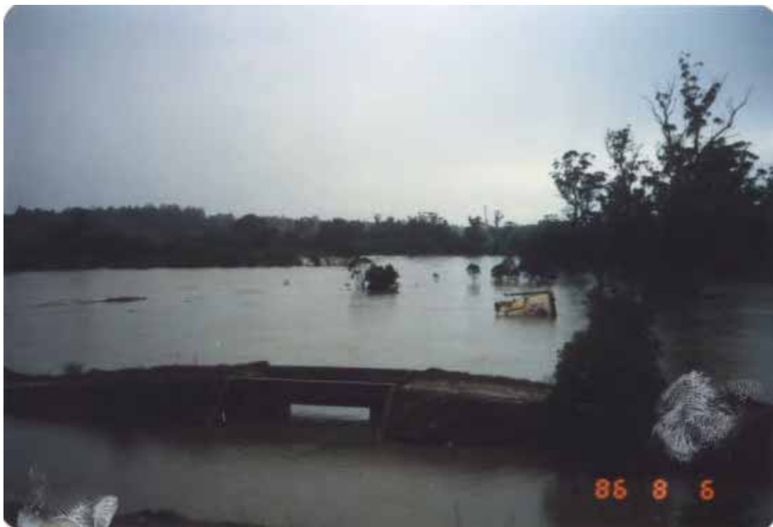
Photo 4 - Flooding of west bank, downstream of Cambridge Avenue (1986 flood)
